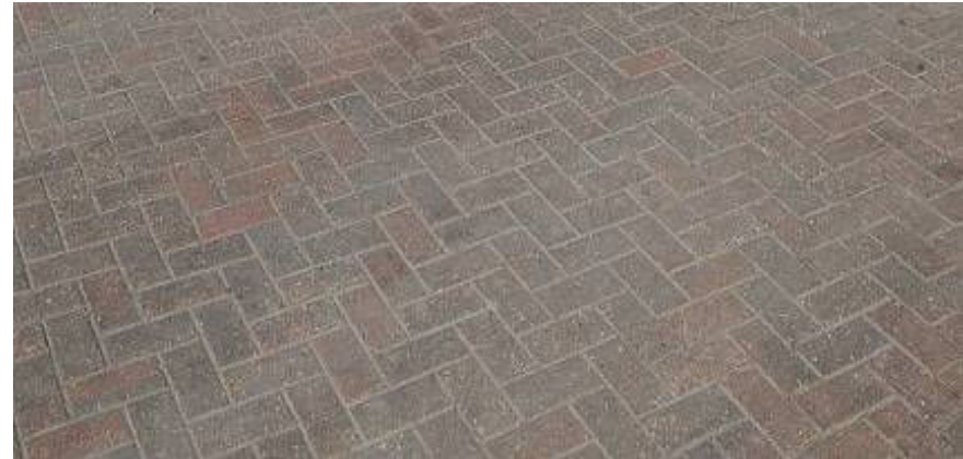
Blocks used on road surface to define a junction at The Parks
