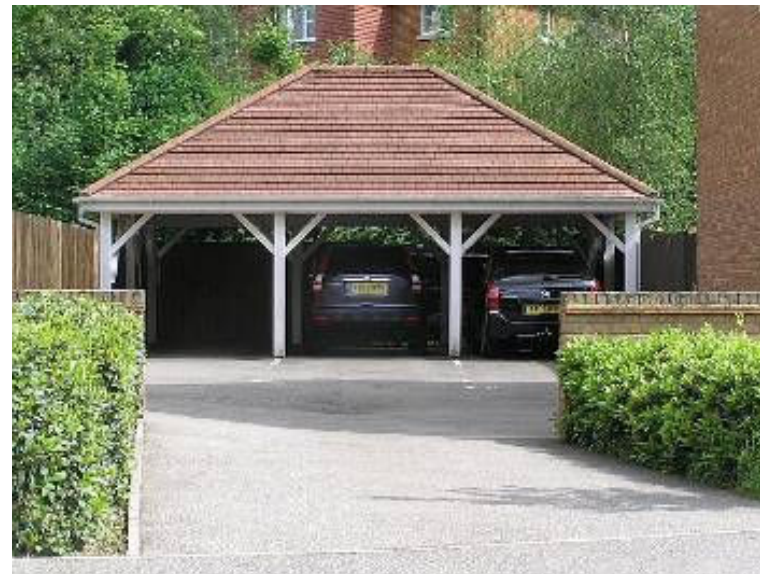
Car barns being used for parking
