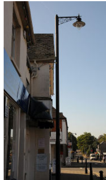
Street lighting designed to inform character
