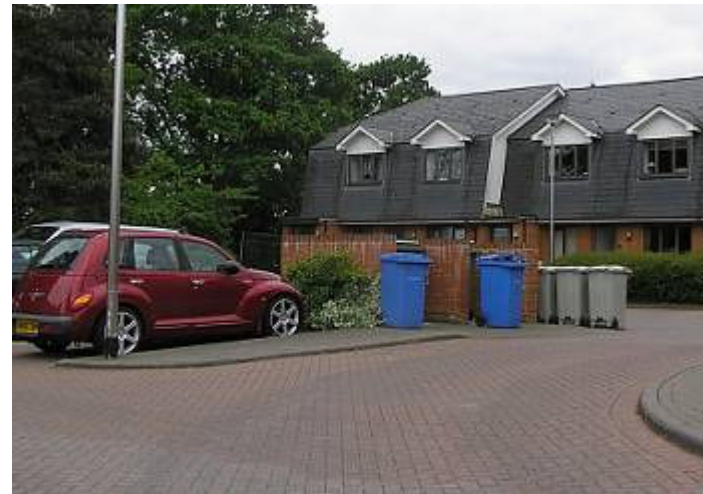
The above bin storage area is visually dominant and poorly screens bins within the streetscene
